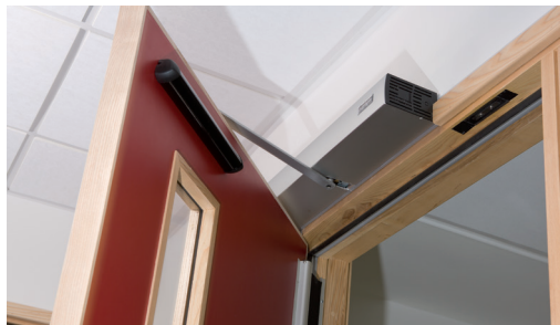
Motion sensor activated power operated door
