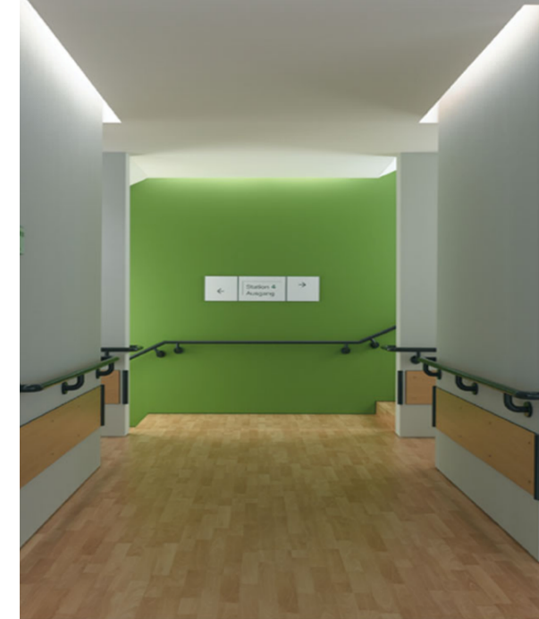
Example of handrails with good visual contrast
